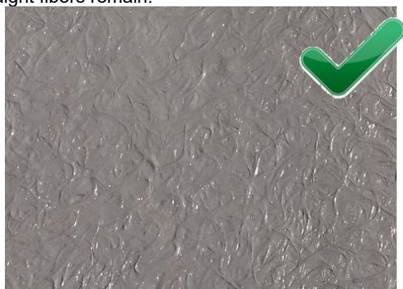
Basecoat applied at correct coverage with matting fully consolidated and “swirly” appearance.
