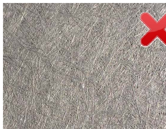
Resin basecoat with under saturated and underworked matting.
